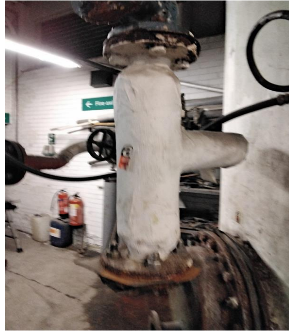
Lagged Pipework
