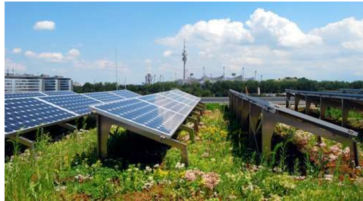
Example of PV roof array
